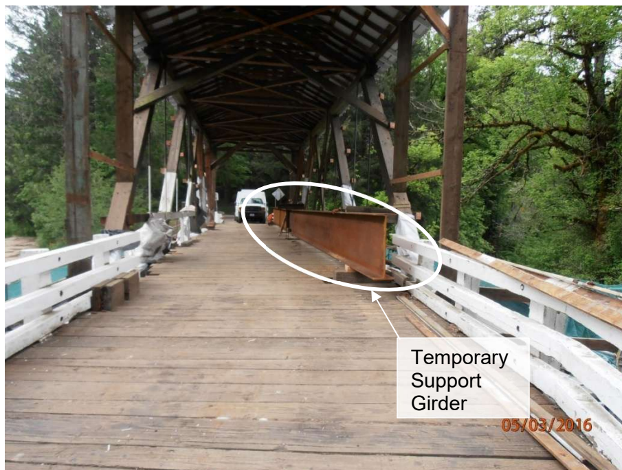
Figure 3: Truss Temporary Support Steel Girder (Wildcat Covered Bridge, 2016)
